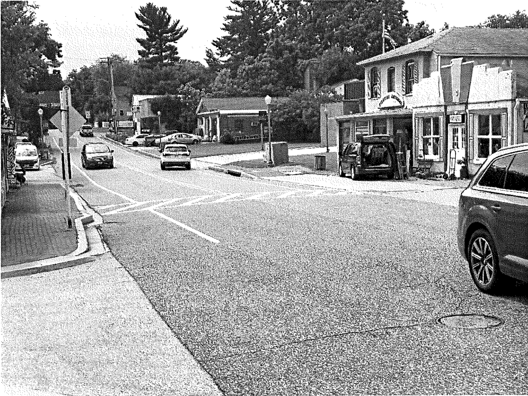
Figure 1: Lanham Severn Road - Looking West
