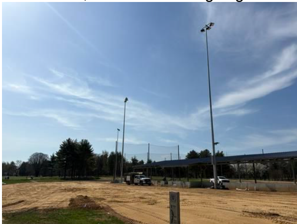
Photo (3/31/26): Stadium lighting installation complete.
