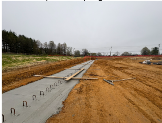
Photo (4/2/26): Concrete footers being placed for the new ice rink foundation.
