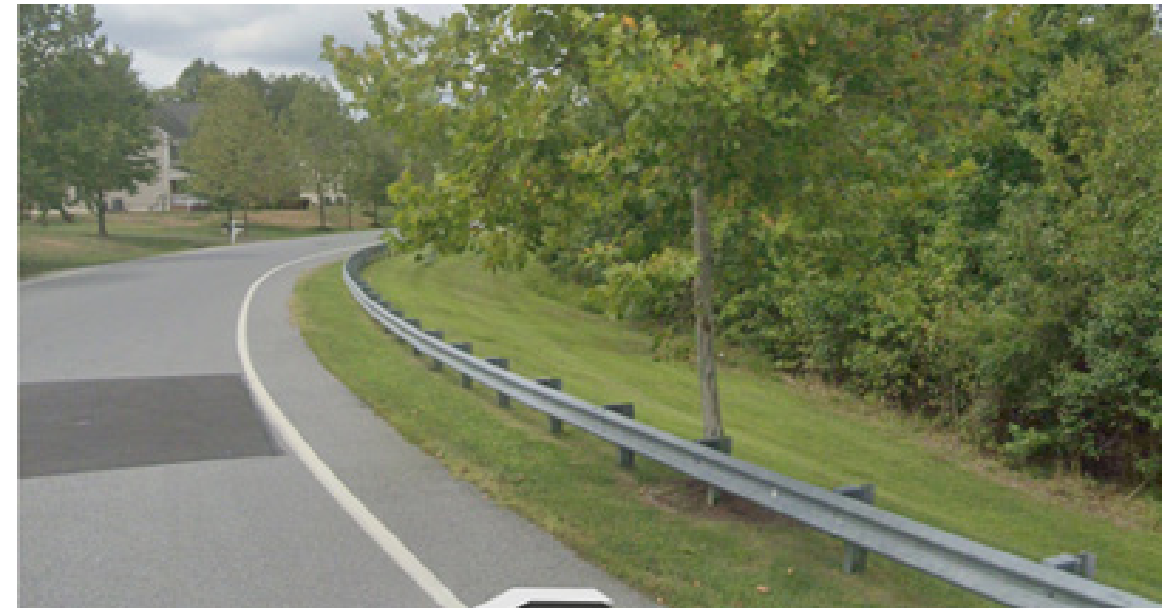
c Existing guardrail looking west along Dahlia Drive. (Source: Google Earth)
