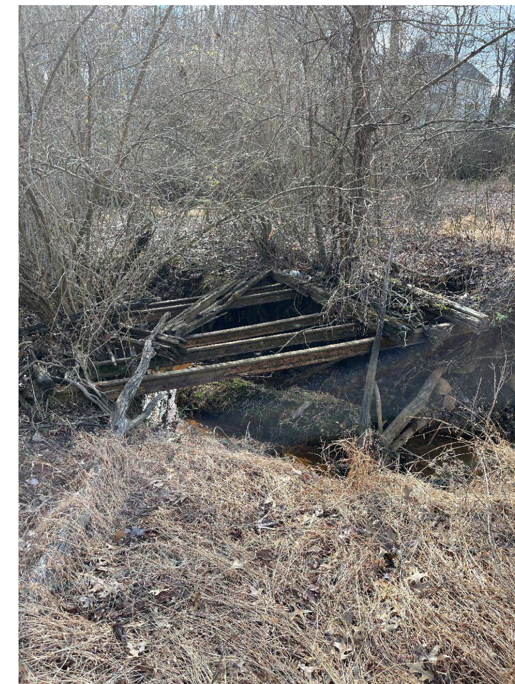
Scrap rail tracks used to support bridge along farm road at proposed stream crossing
