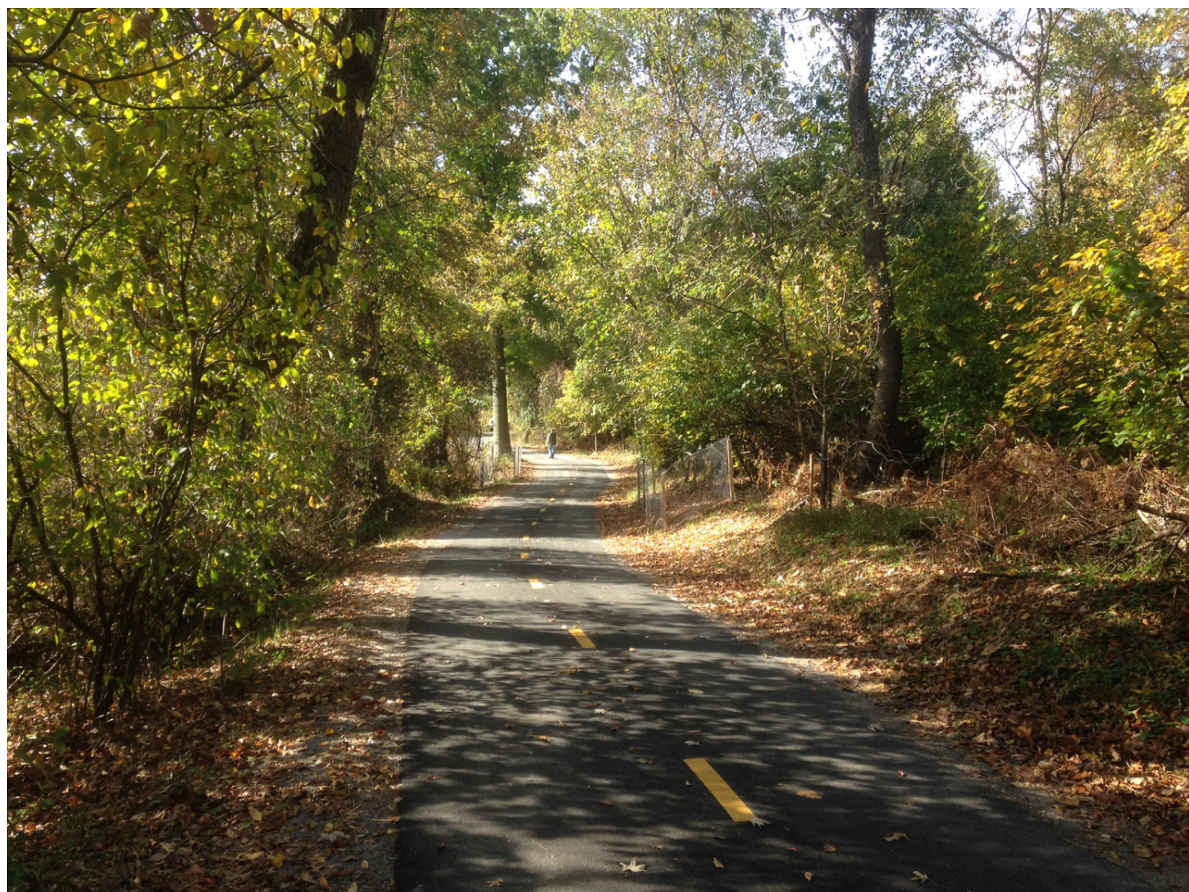
Example of ten-foot paved multi-use pathway (Anacostia River Trail near Kenilworth Aquatic Gardens)
