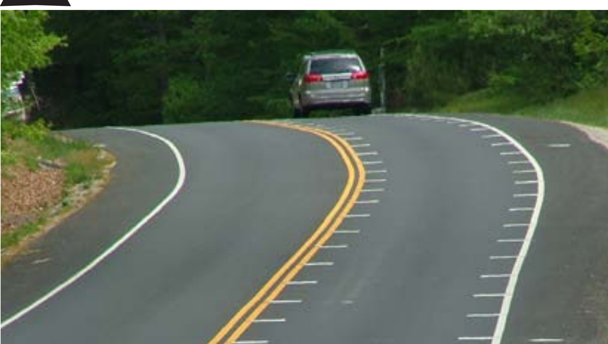
Transverse edge striping (courtesy of VDOT)
