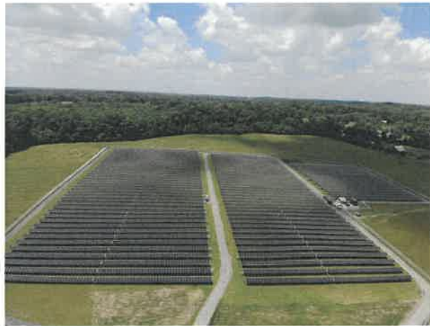
A photo of the City's solar farm.
