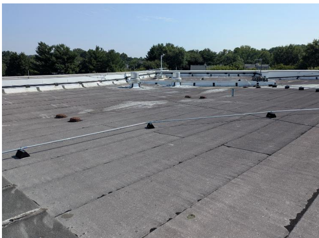
Figure 30: Existing roof at City Hall
