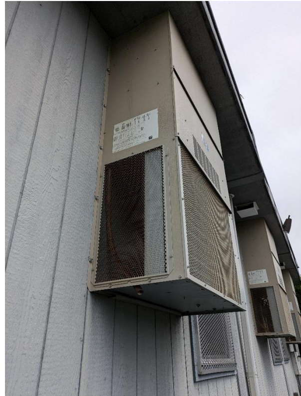
Figure 10: One of three food pantry trailer PTACs
