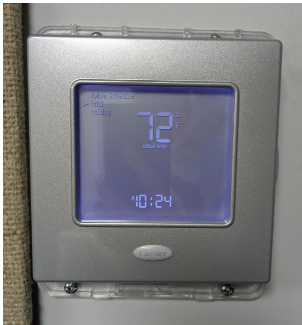
Figure 28: Typical programmable thermostat at Kenhill Center with “hold” selected
