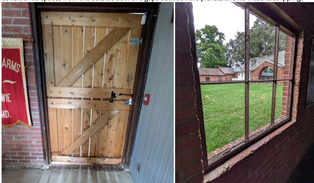
Figure 51: Barn door and window at Belair Stables
