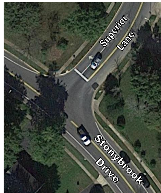
Figure 1: Aerial of Study Intersection
