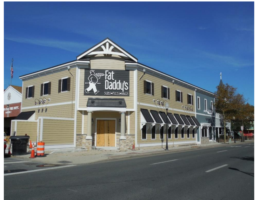
Construction in Progress
